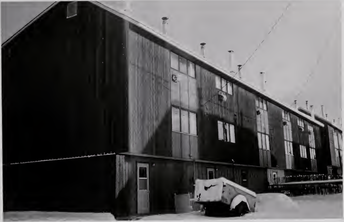
Plate 12. Maisonettes in Faro. The object beneath the upstairs window is a rope ladder to be used in case of fire. (December 4, 1971).
